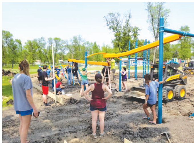
The community build project installing new play equipment.
